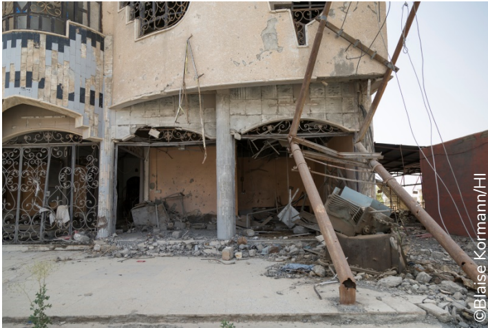
Destruction to a home in Hamdaniya, Iraq
